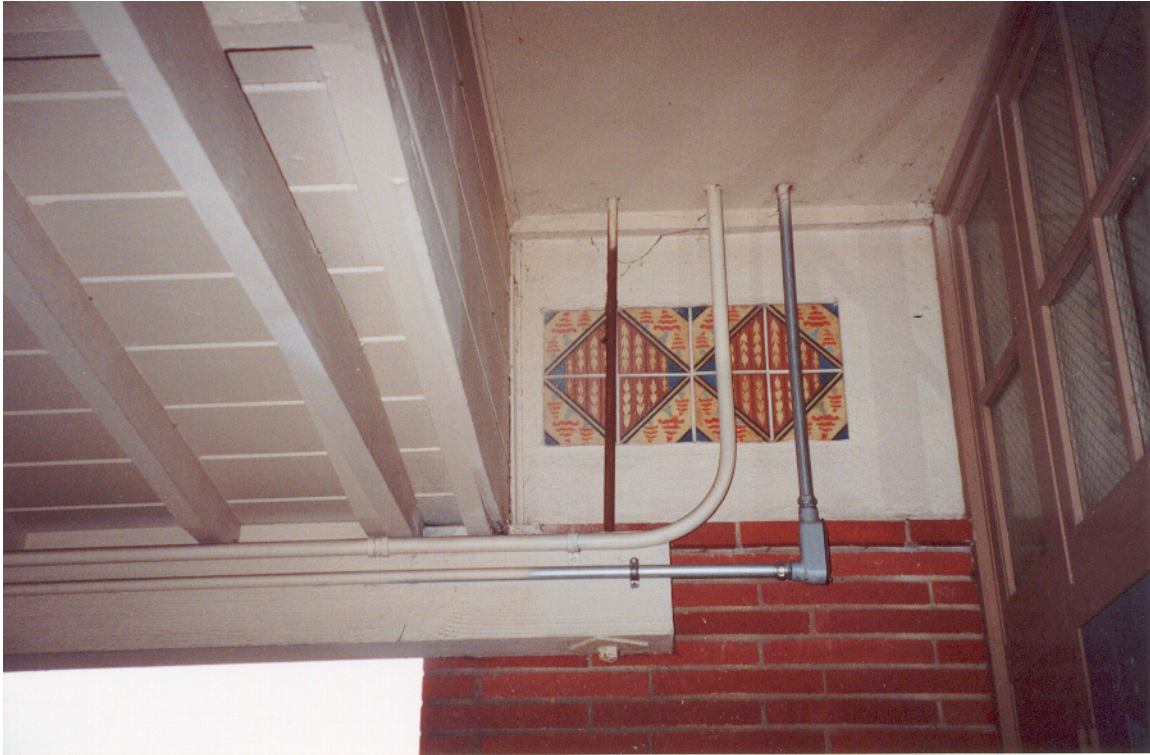
Figure 12: Hanger rods at covered walkway
