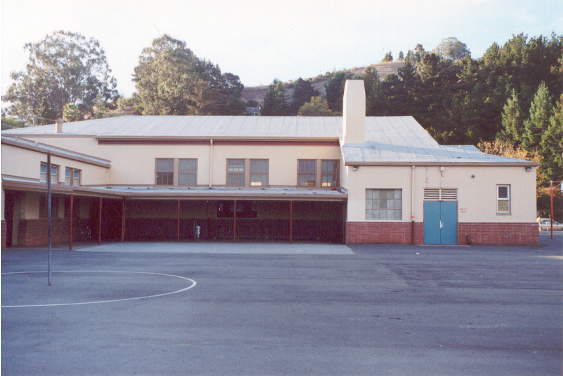
Figure 5: Main building and auditorium
