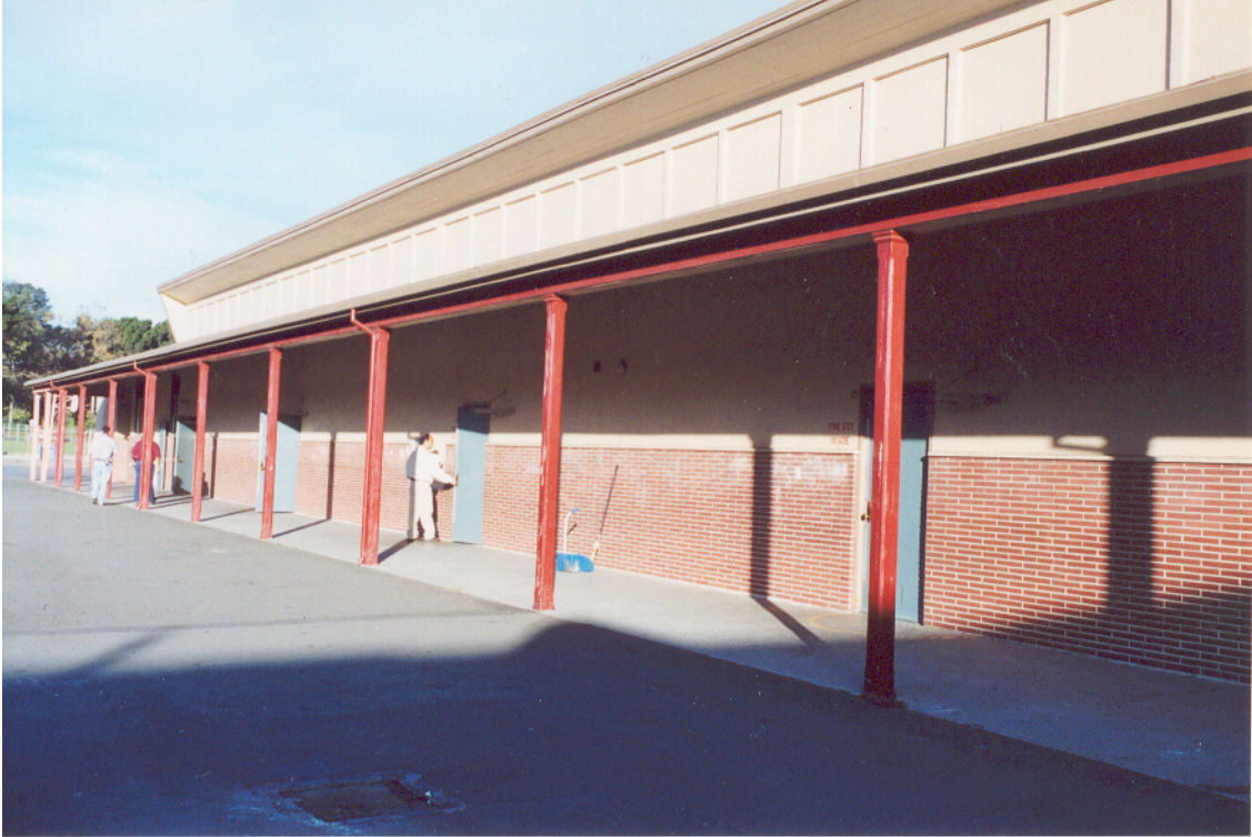
Figure 6: Classroom building, rooms 10-13 (south face)
