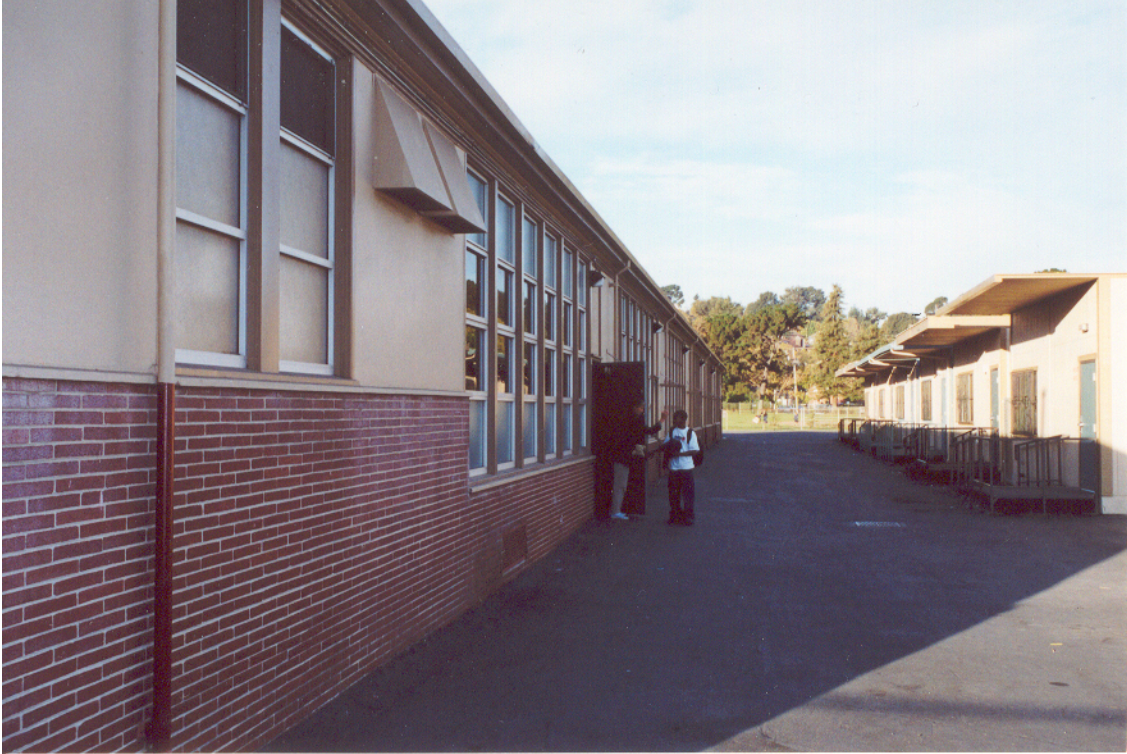
Figure 7: Classroom building, rooms 14-19 (north face)
