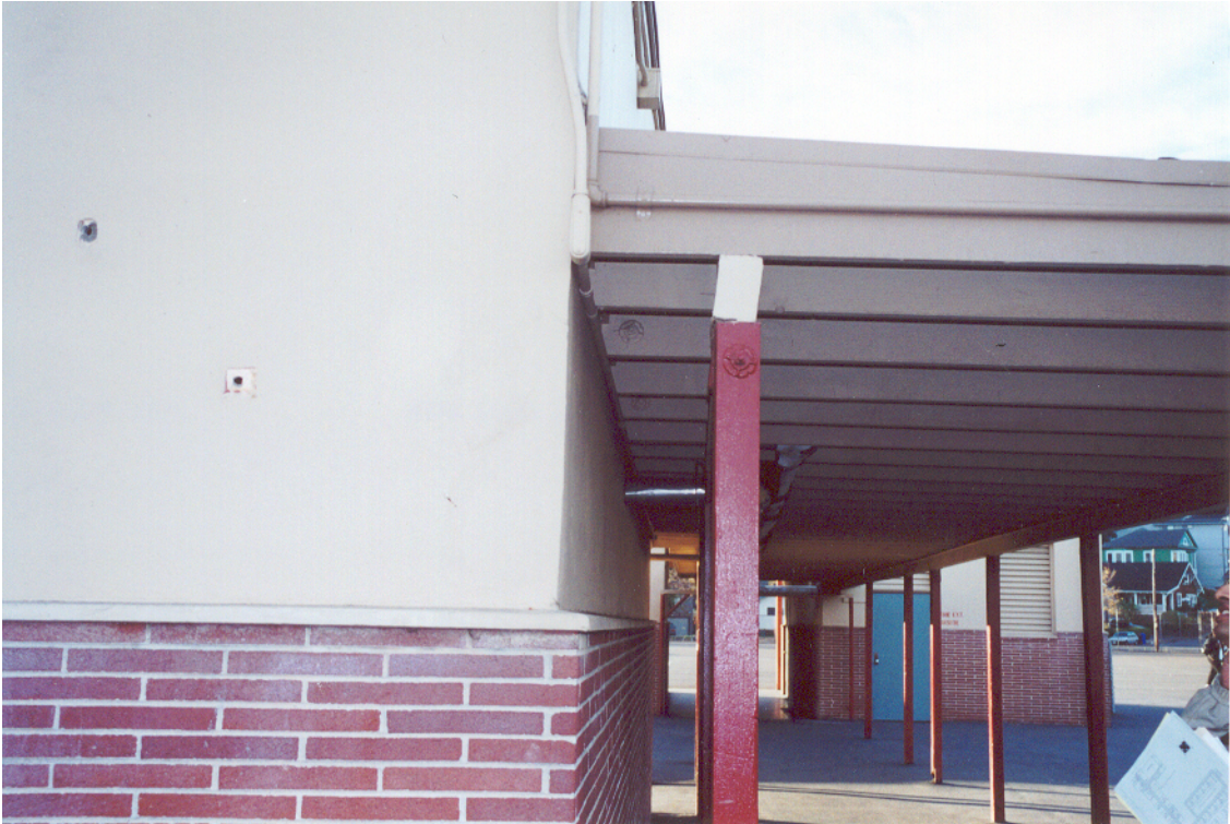
Figure 11: Covered walkway at classroom building (near room 19)
