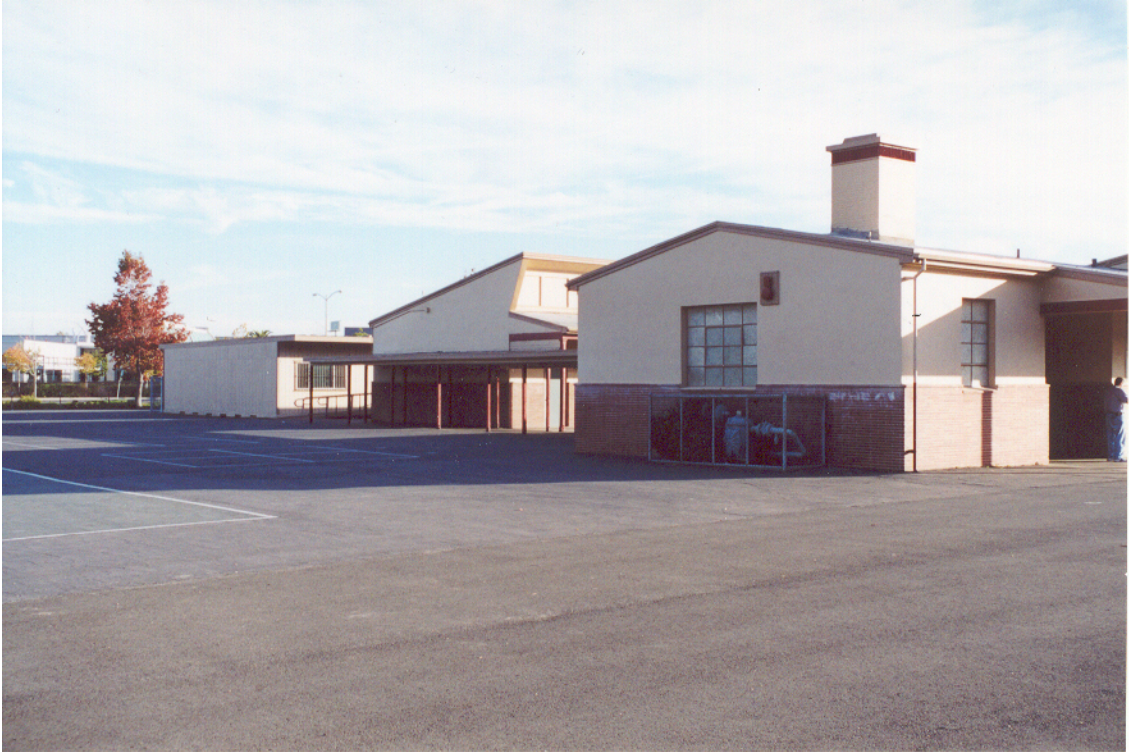
Figure 8: Classroom buildings (west side)
