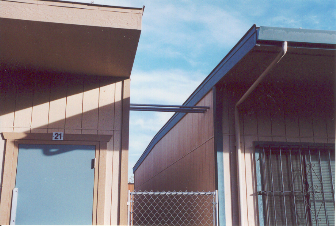
Figure 13: Electrical conduit at portables
