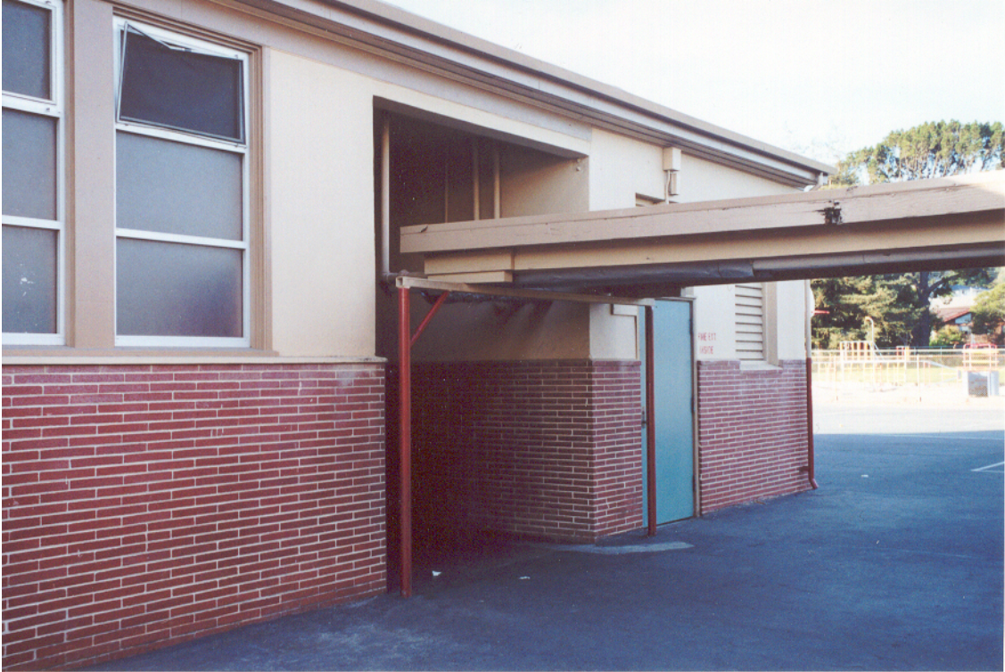
Figure 10: Covered walkway at classroom building (near room 13)
